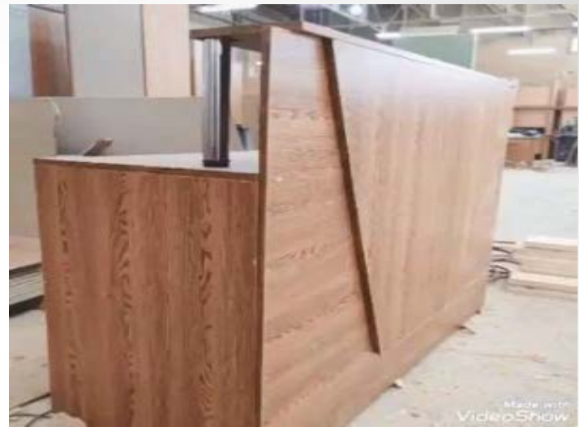
installation of reception counters
